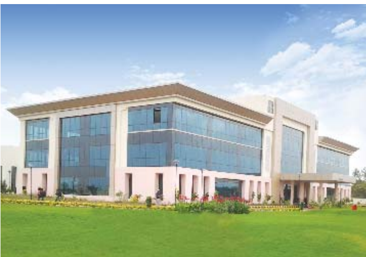
Switchgear Factory, Vadodara
