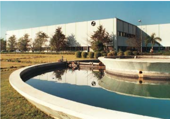
Switchgear Factory, Ahmednagar
