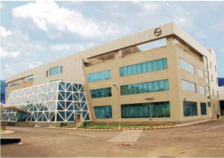
Switchgear Factory, Navi Mumbai
